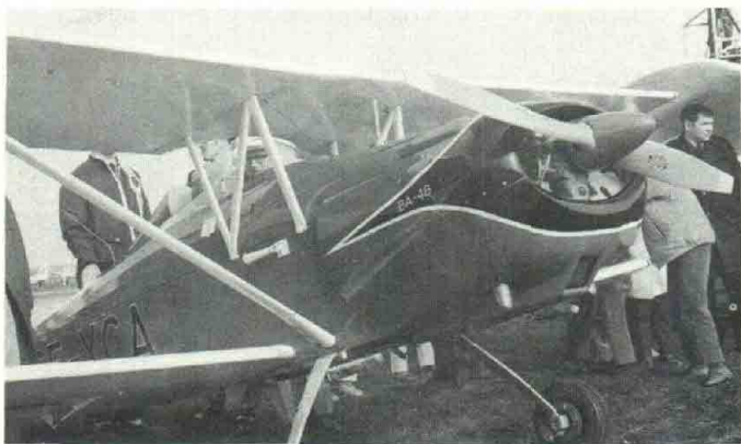
Tage Simonson's Andreasson BA-4B, SE-XCA, won the best-workmanship award. Wood and fabric wings are employed rather than the standard all-metal wings for this type.
