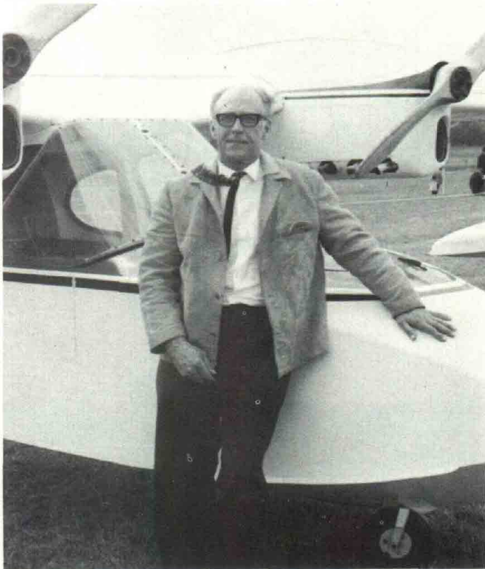
This handsome German-registered amphibian was built by Carl Johannsen of Denmark. Power is two 65 hp Walter "Mikron III" engines, the wing is full cantilever, and the airplane is generally quite clean. The main gear legs swing upward and slide inward for flush retraction. The builder poses with his amphibian which is much smaller than one would expect.
