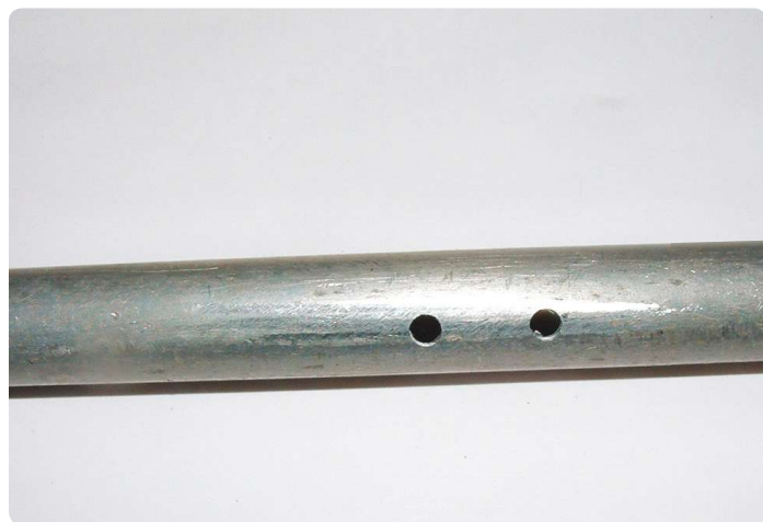
These photos show vent holes drilled in longerons and diagonals as they would form a cluster over the vent holes. Holes allow both venting and oil flow.
