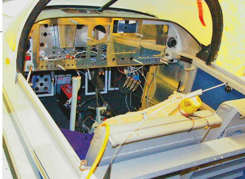
The panel in mid remodel.
