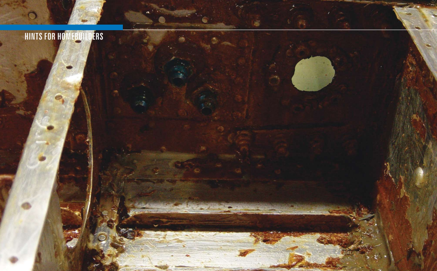
1. Initial progress ... we have access to the tank.
